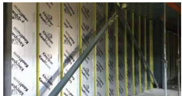
Figure 6 Side elevation of Kingspan Kooltherm ® K12 Framing Board clip-and-channel system
